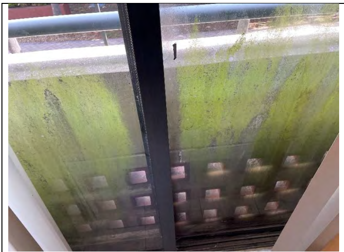
11. View of typical water exposure and algae buildup on exterior sliding door in PEI 212
