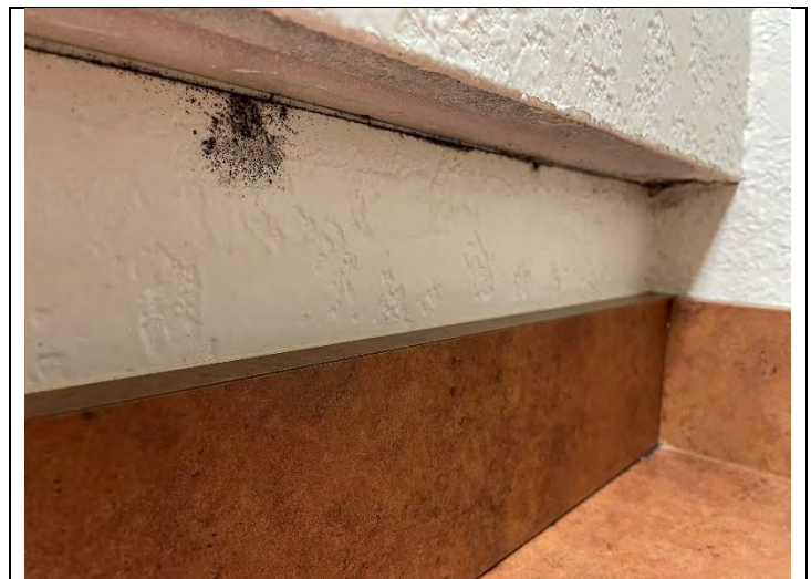
40. View of SVG under restroom mirror PEI 331
