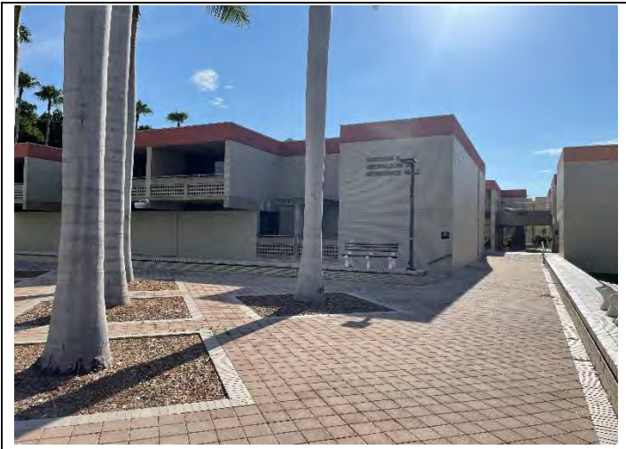
1. View of PEI 2 Building (exterior)
